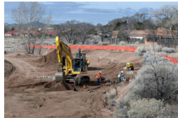
Heavy equipment is part of the artillery in a city project to install erosion
