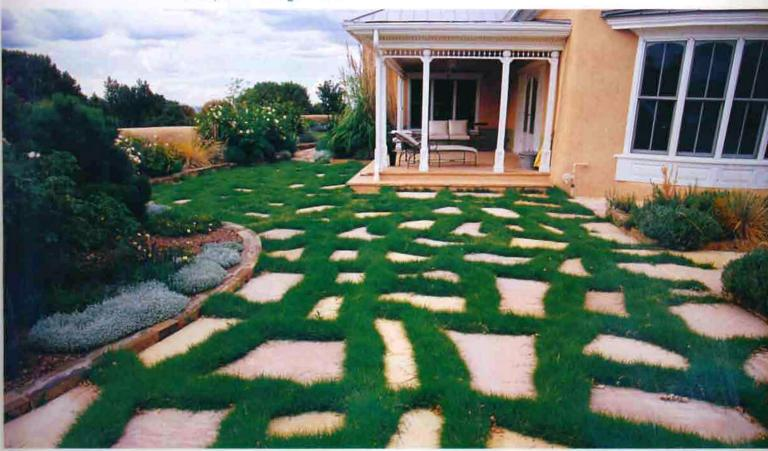
Capture rainwater ranoff by creating wicks of purilice under flagstones, with native grass growing in the wide seams. The flagstones keep the lightweight purilice from floating when the wicks fill with rain and capture condensation to support the grasses (Garden design by Santa Fe Permaculture).
